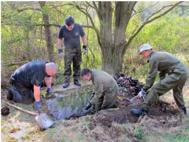
Excavating Insulators from Cable Entry Shaft 1. Photo Clive Penfold
